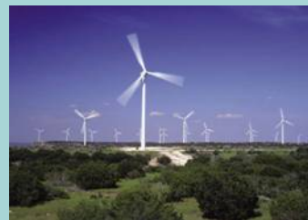
Courtesy of General Electric
